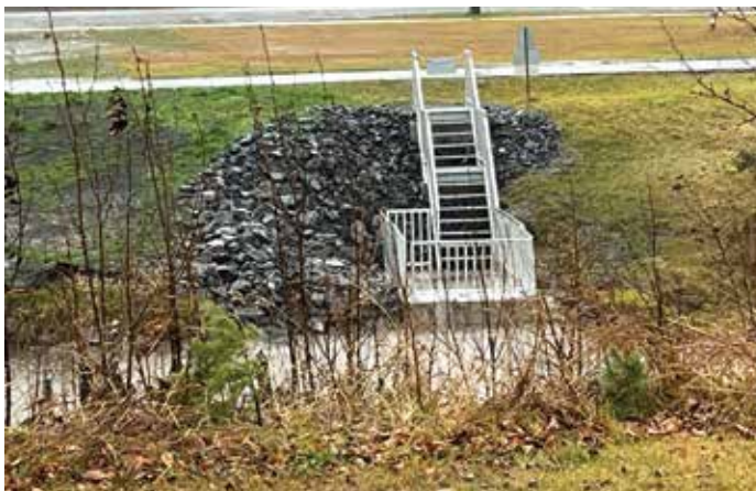
New lamprey trap installation on the Neebing River—2024
