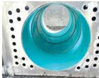
Counter tubes determine numbers as well as ease migration of fish entering the fishway.
