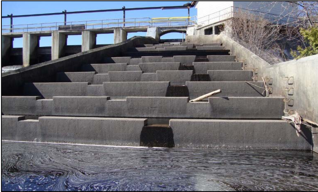
Figure 2-4. Photograph looking upstream showing the fishway weirs and notches without flow (Source: https://northshoresteelhead.com/project/current-river/fishway-project/gal )
